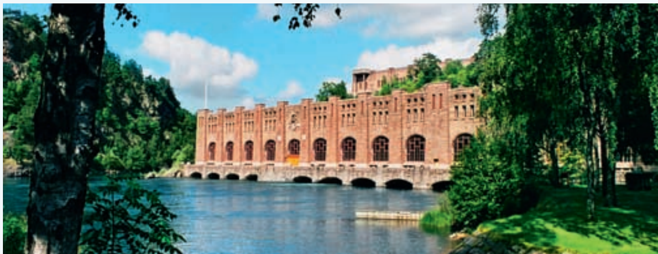
Olidan, on the Göta River, was one of the first hydro power stations built between 1909 and 1916 by the newly formed Swedish State Power Board.
